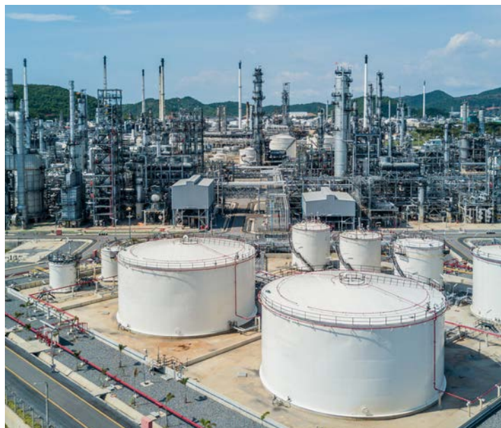
Large-scale oil refinery developments are expected to remain a key driver of project cargo demand across Africa over the coming years.
