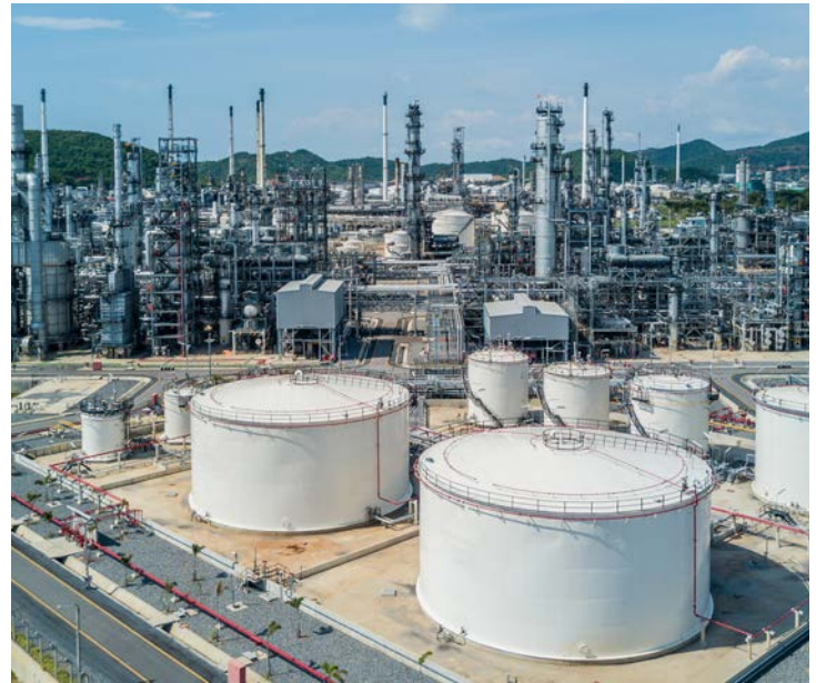
Large-scale oil refinery developments are expected to remain a key driver of project cargo demand across Africa over the coming years.
